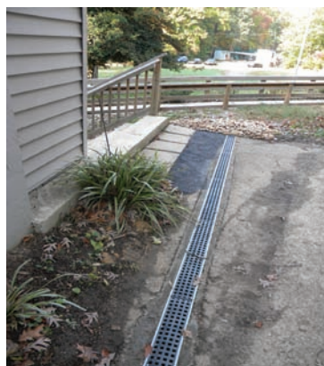
New channel drain to stop runoff from the parking lot.
